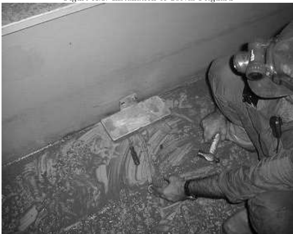
Figure A.1: Installation of Tsevas Pitguard
