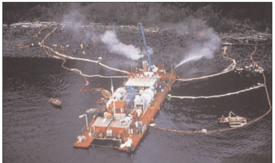
Hot water washing of a beach in Prince William Sound, Alaska, that had been oiled by the Exxon Valdez spill in 1989. Much of the shore life could not survive temperatures that reached 60°C.
